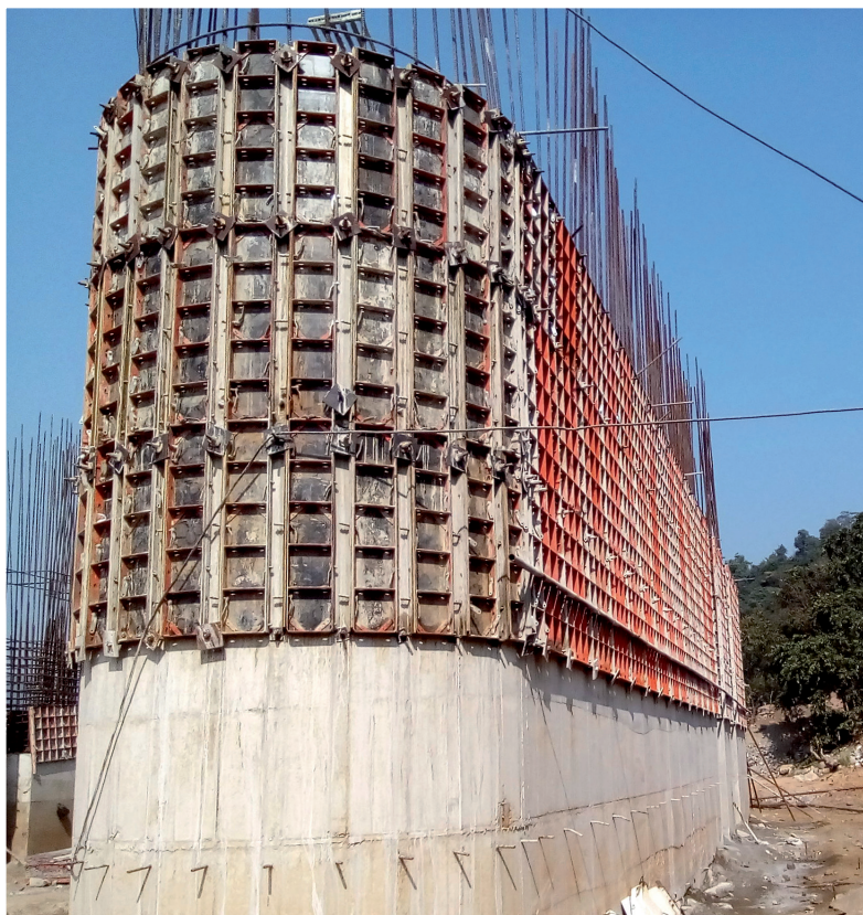
Shuttering height of up to 3.75 m reached with three element heights of 1.25 m each. The semi-rounded formwork unit was custom made by PASCHAL Formwork (India) Pvt. Ltd. for the construction company M / S. Baitarani Power Project Private Limited.
