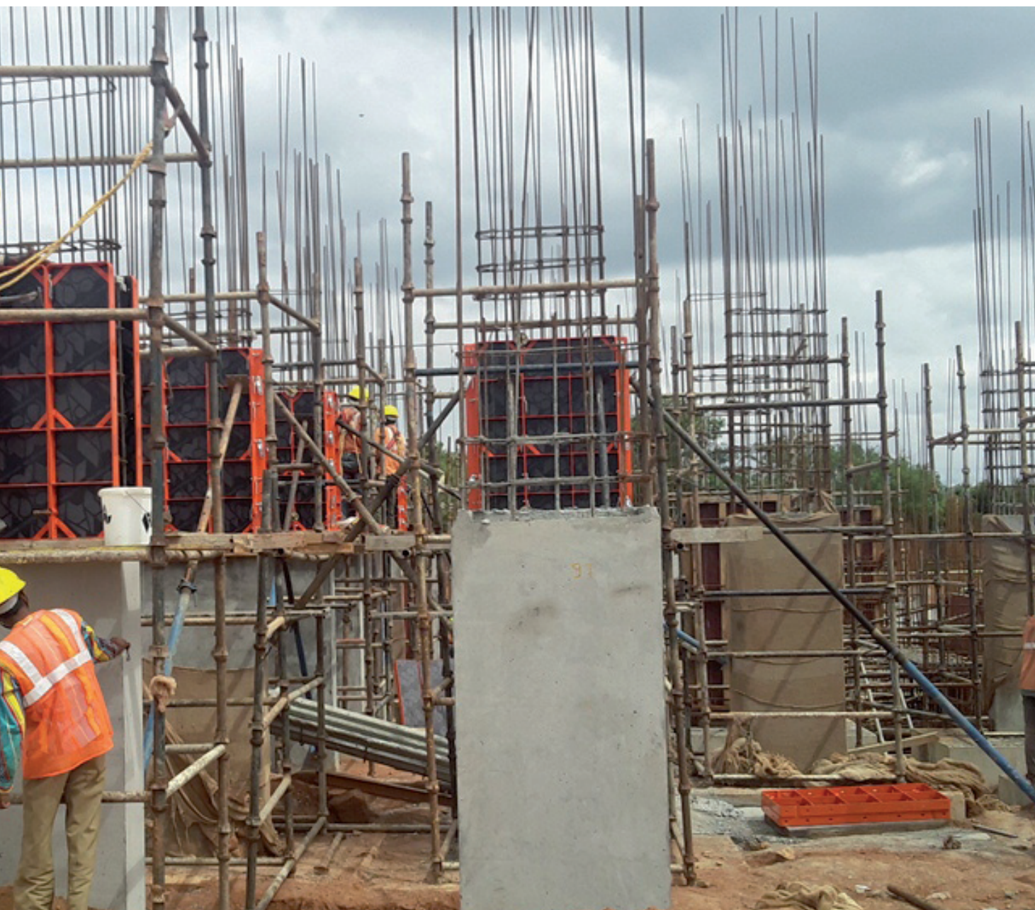
With the Modular elements, formwork will be provided for over 50,000 m 2 to build another dam in India
