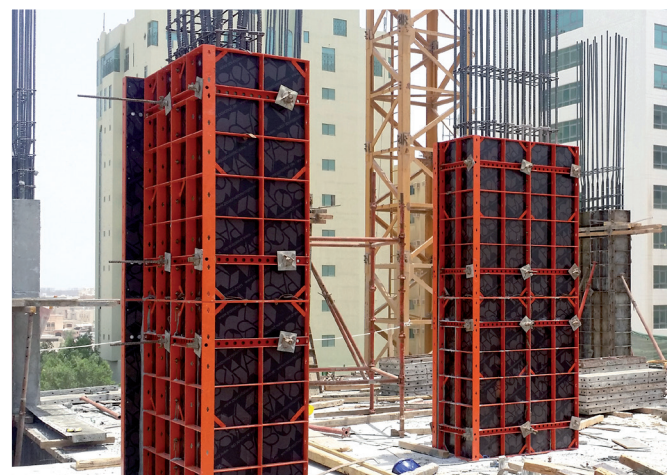
The adjustable Modular column formwork in practical use.
