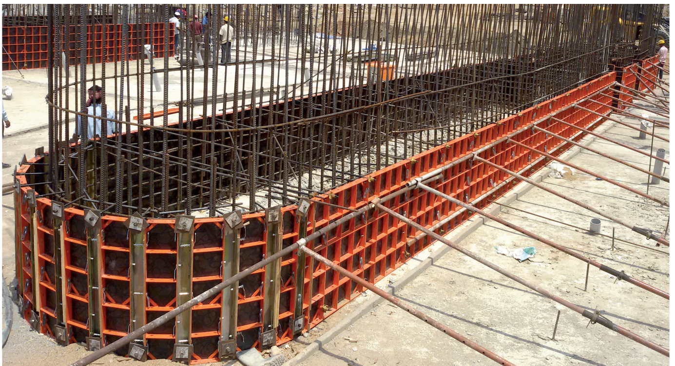
With the Modular elements, formwork will be provided for over 50,000 m 2 to build another dam in India
