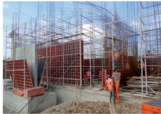
Modular universal formwork on a building site in India.
