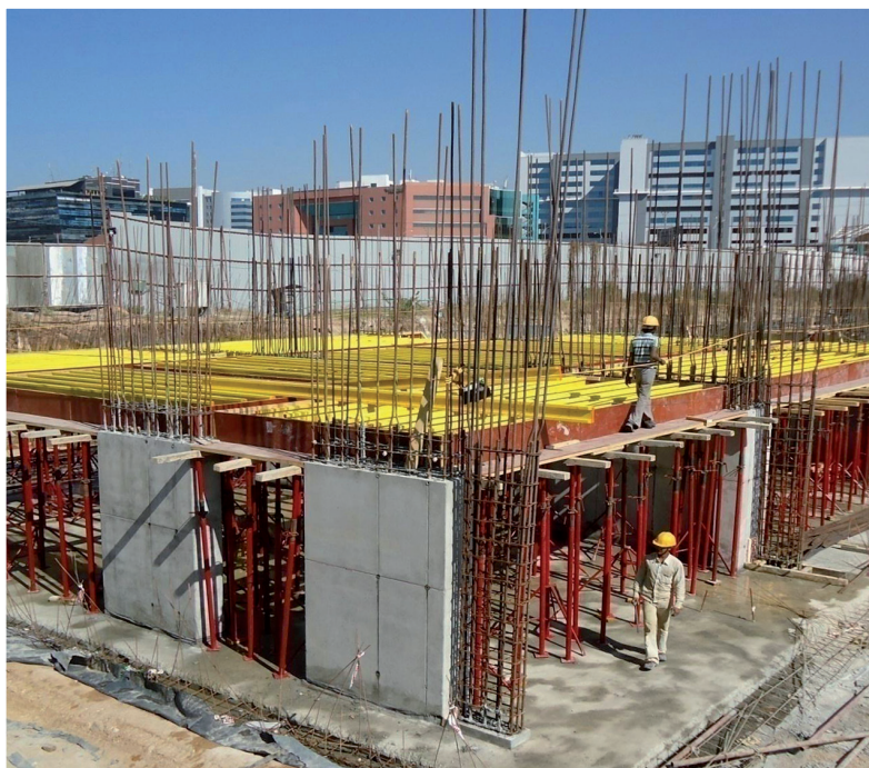
PASCHAL Deck - versatile slab formwork for ceilings in residential and industrial buildings.
